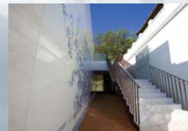
A new building in the precincts of Kotohira Shrine designed by the author
