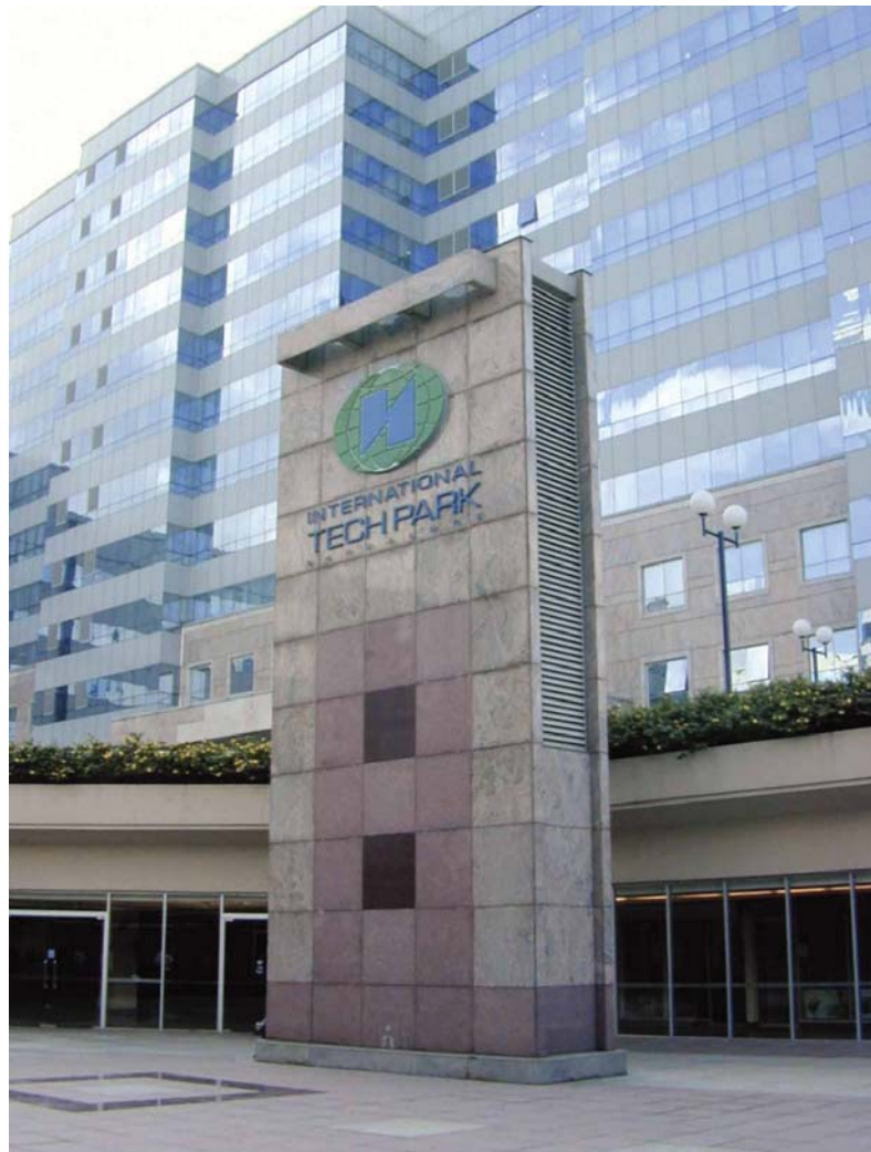
An IT industrial complex in Bangalore
