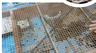
Making seed balls by using sieves for construction
