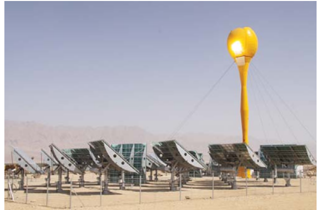
Aora's solar energy site at Kibbutz Samar
