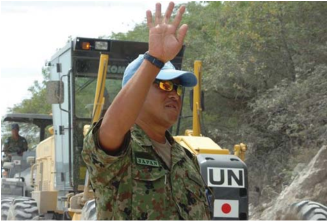
Road repair by Japanese Self-Defense Forces troops near Haiti-Dominican Republic boarder
