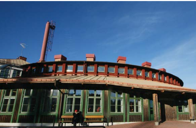
Heating and cooling at Lagggarberg, inspired by the termites
