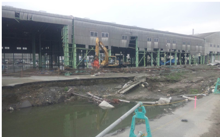
Paper mill in industrial zone in coastal part in Ishinomaki
