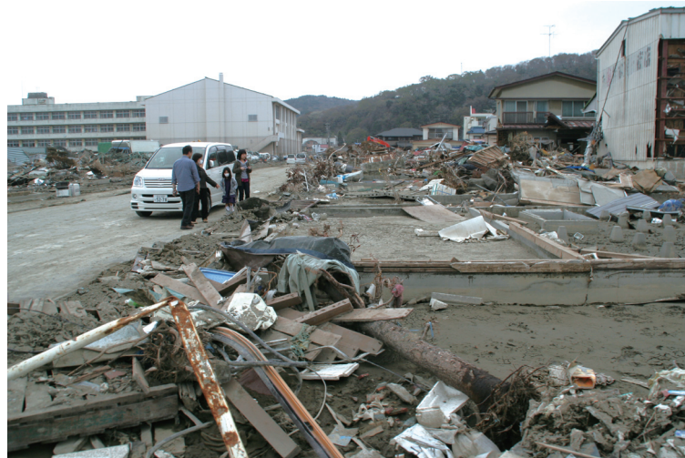
Ishinomaki City, where about 80% of offices were damaged by the tsunami
