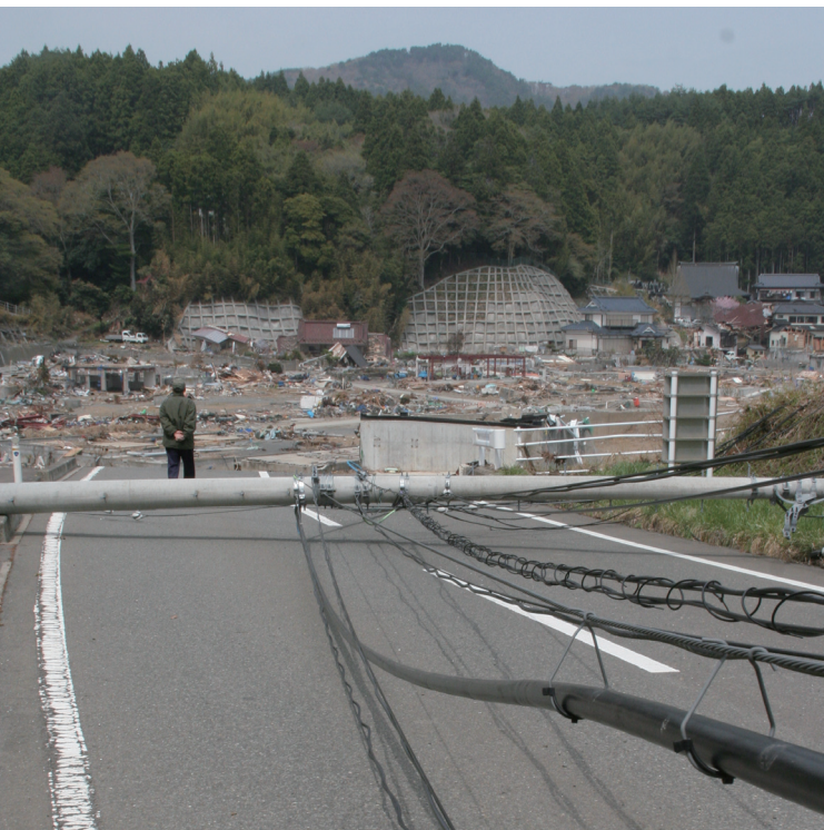
On this side of the man, the road is blocked by a power pole; on the other, it has collapsed.
