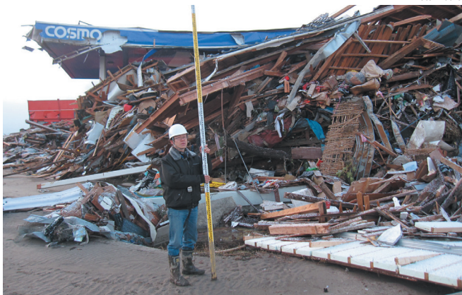
Tsunami damage to buildings along the coast (Sendai).
