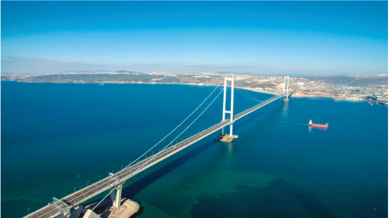
Osman Gazi Bridge (Izmit Bay Crossing Bridge) in Turkey, the longest suspension bridge in the country, which opened in 2016.
