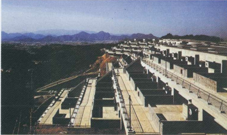
An application of the Stratiform Structure System to apartment housing in Shizuoka, Japan
