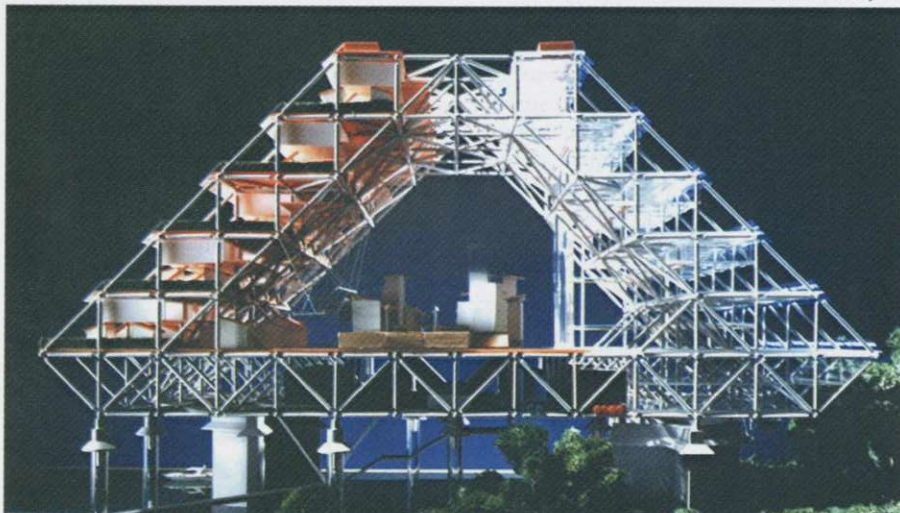
The Stratiform Structure System can be disassembled and reassembled with a triangular-shaped structure that can withstand earthquakes and typhoons
