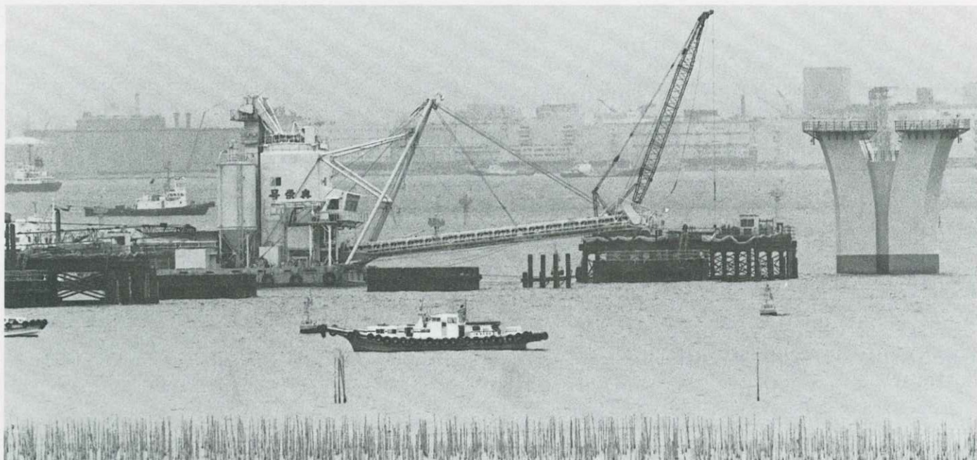
Trans-Tokyo Bay bridge construction—the largest public works project in fiscal 1992.
