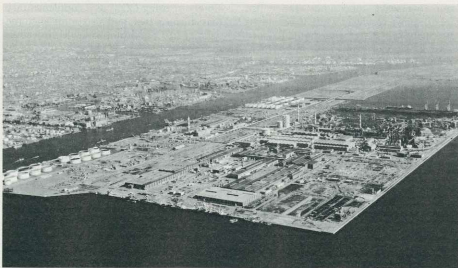
Aerial view of the Ohgishima complex that has an annual crude steel processing capacity of 6,000,000 tons.
