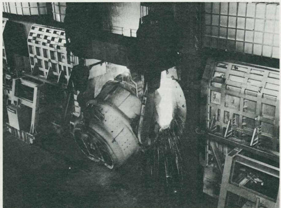
Bottom blown converter (Q-BOP) was introduced for the first time in 1977 by Kawasaki Steel.
