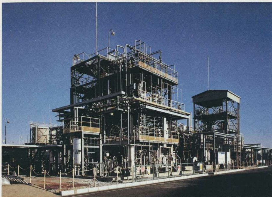
One-ton/day process development unit for coal liquefaction
