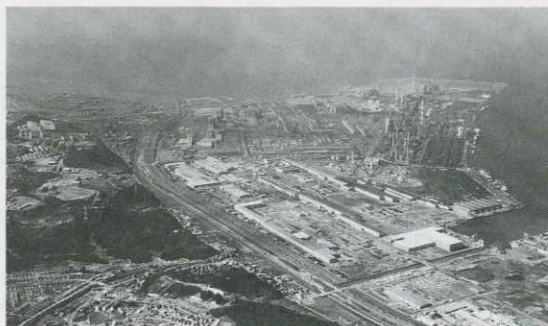
Decreased domestic demand in steel industry inevitable. (Nippon Steel Corp. Kimitsu Ironworks)
