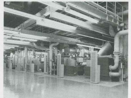
An energy-saving heat pump that turns exhaust heat into new heat energy. Various factors are pushing Japan to further examine its long-term energy policy.
