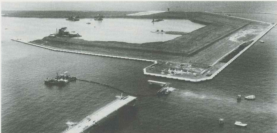
Construction work continues on the New Kansai International Airport. Its opening has been put back by over a year to the summer of 1994 due to the sinking of reclaimed land.
