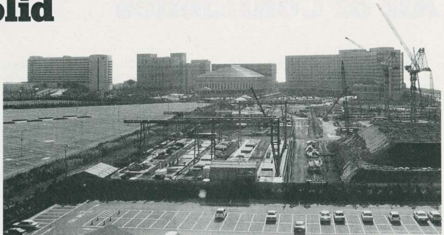
Construction companies' revenues and profits will continue growing in the year ahead.
