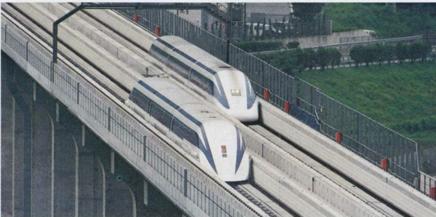
Photo 3: To test safety and stability, two trains were operated in parallel lanes at a relative speed of 1003km/h
