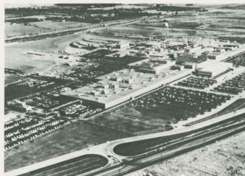
Toyota plans to produce 200,000 subcompacts annually with GM at the NUMMI plant in Fremont, California.
