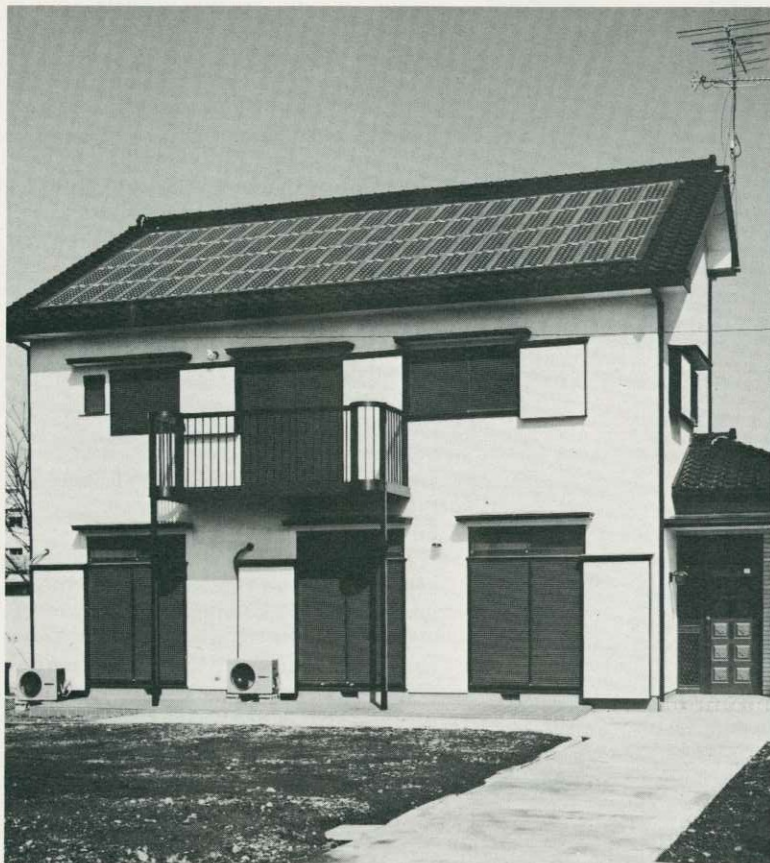
NEDO experimental house in Yokosuka, Kanagawa Pref., with photovoltaic power system
