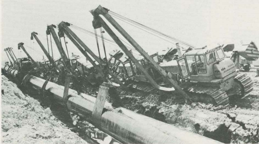
The tubes for the natural gas pipeline being laid near Shgorod, west of the Ural mountains. Japan buys a large amount of natural gas from the Soviet Union.
