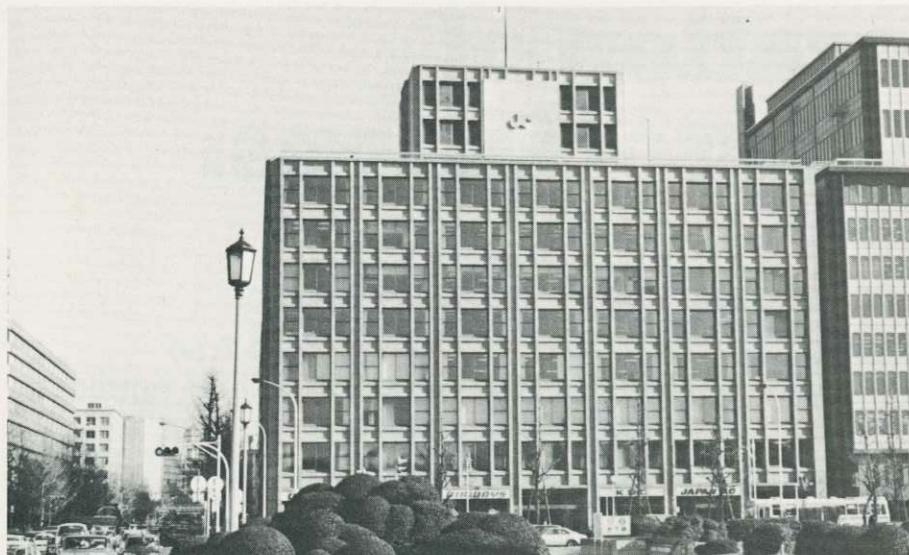
The Tocho building which houses Nissho headquarters.
