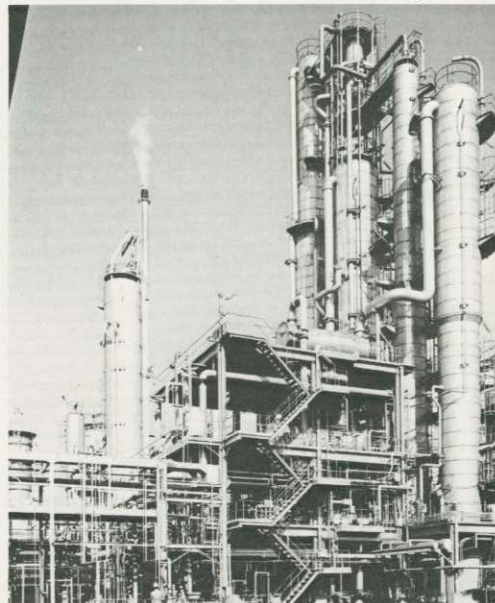
Asahi Chemical's ammonia plant in Mizushima, Okayama Pref.
