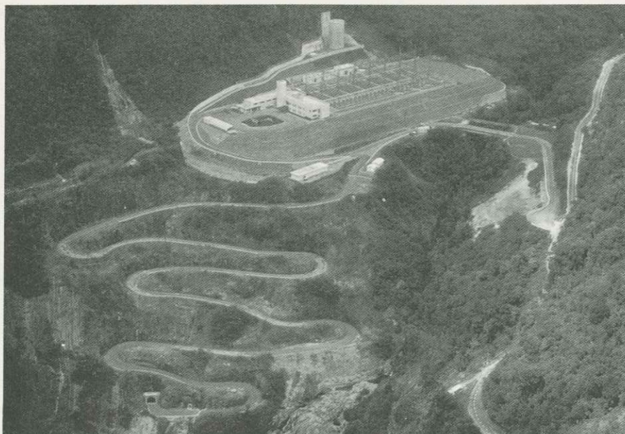
One of the hydroelectric power stations being built as a part of the Asahan Project. One ton of aluminum requires 15,000kWh of electricity to produce.
