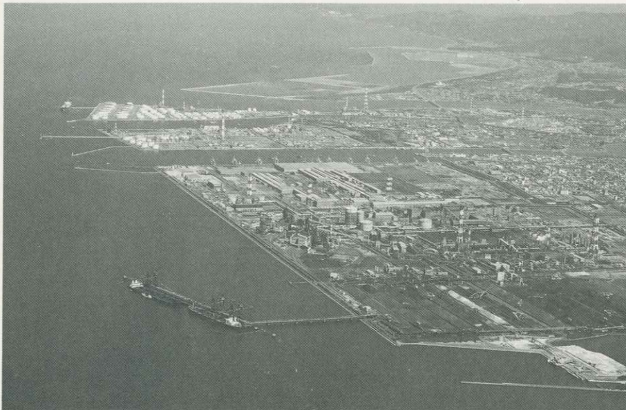
Aerial view of Oita District New Industrial City
