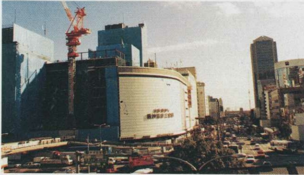
Restoration work in Kobe following last year's disaster.
