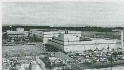
Major steel mills are stepping up their investment in equipment and research and development efforts despite increasing costs.
