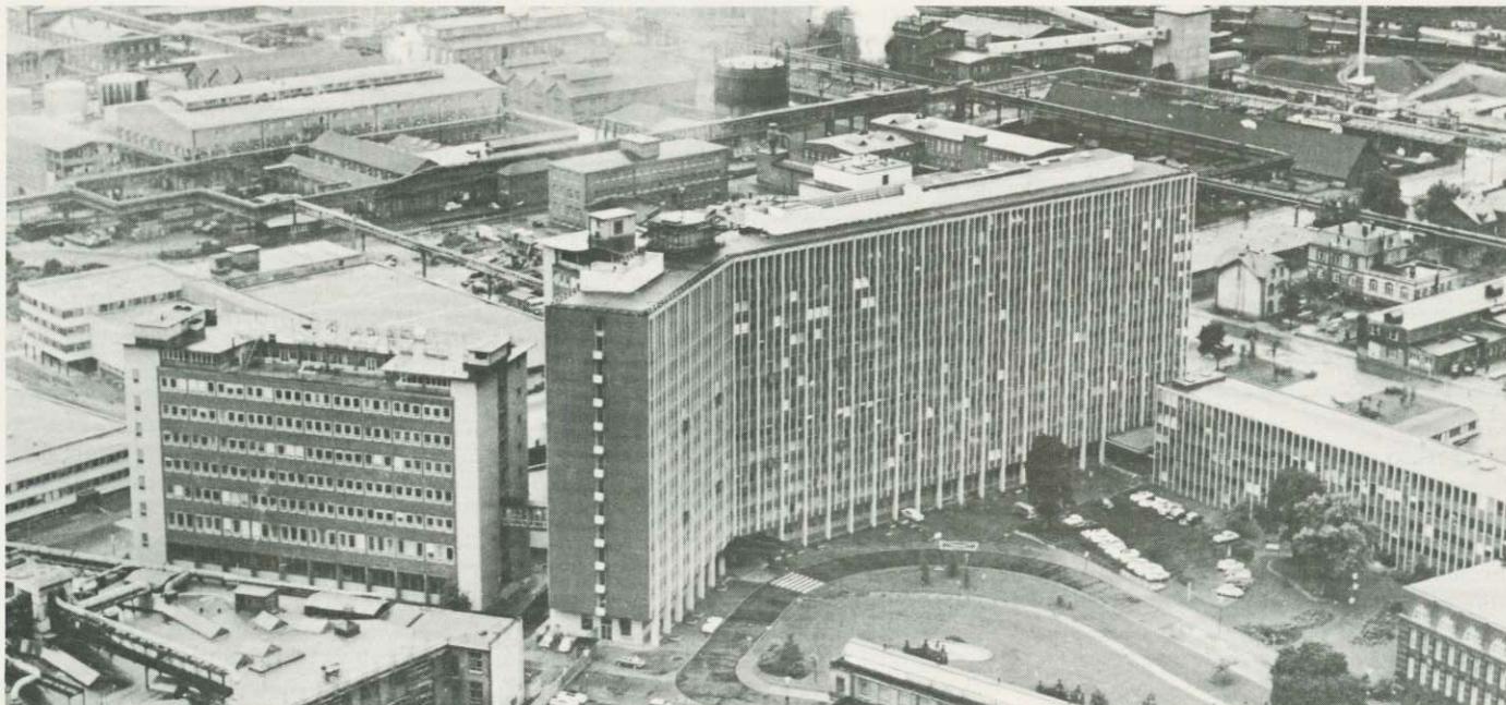
Hoechst's headquarters building in Frankfurt, West Germany
