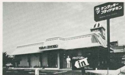
"Drive-through" type shop in Chiba, southeast of Tokyo
