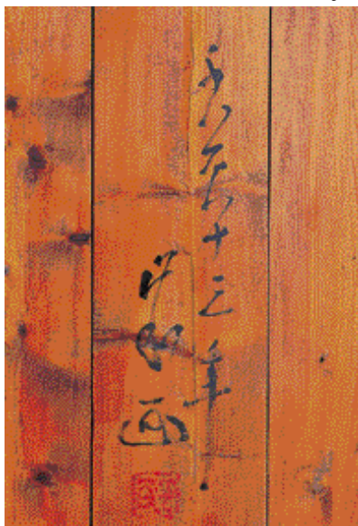
Signature and date written by Yamamoto Hosui on the north wall of the annex
