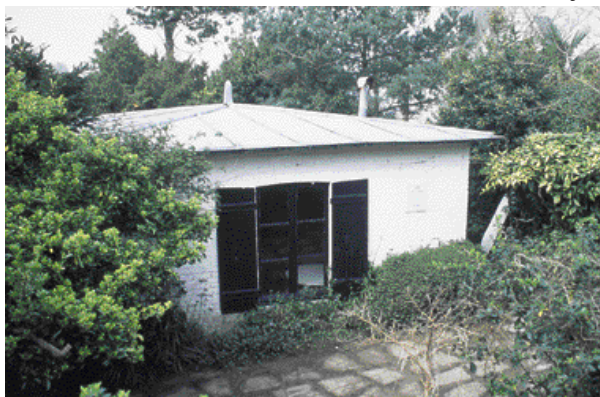
A small annex in the corner of the garden of Pré des Oiseaux
