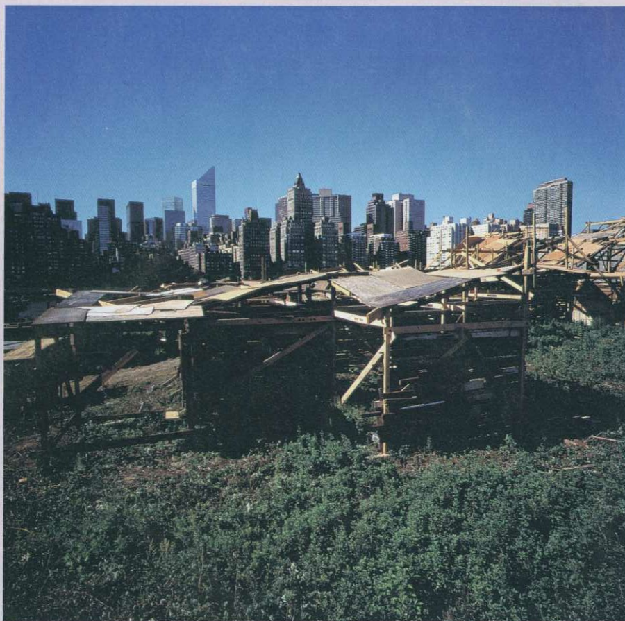
Project on Roosevelt Island New York, 1992/scrap (wood, metal, etc.) by Kawamata Tadashi. Photo: Kashiwagi Hisayasu. ©Kawamata + on the table, Tokyo.
