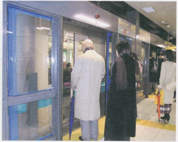
All platforms of the Nanboku Line subway are enclosed with walls and gates
