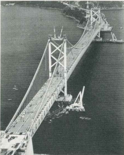
The Ohnaruto Bridge connecting the main Japanese island of Honshu with Shikoku is a typical example of a government public project incorporating private-sector expertise.
