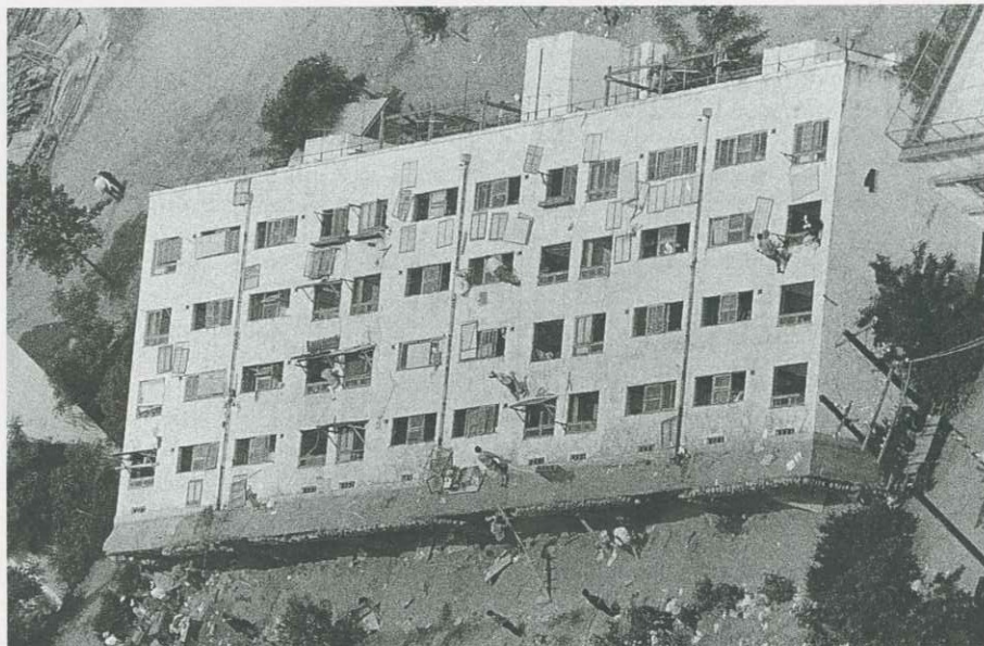
An apartment building that was literally knocked over by a large earthquake near the city of Niigata in 1964.
