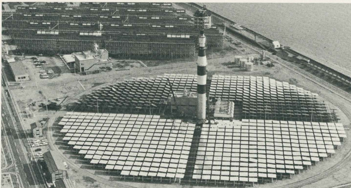
Solar power generating plant in Shikoku, Japan
