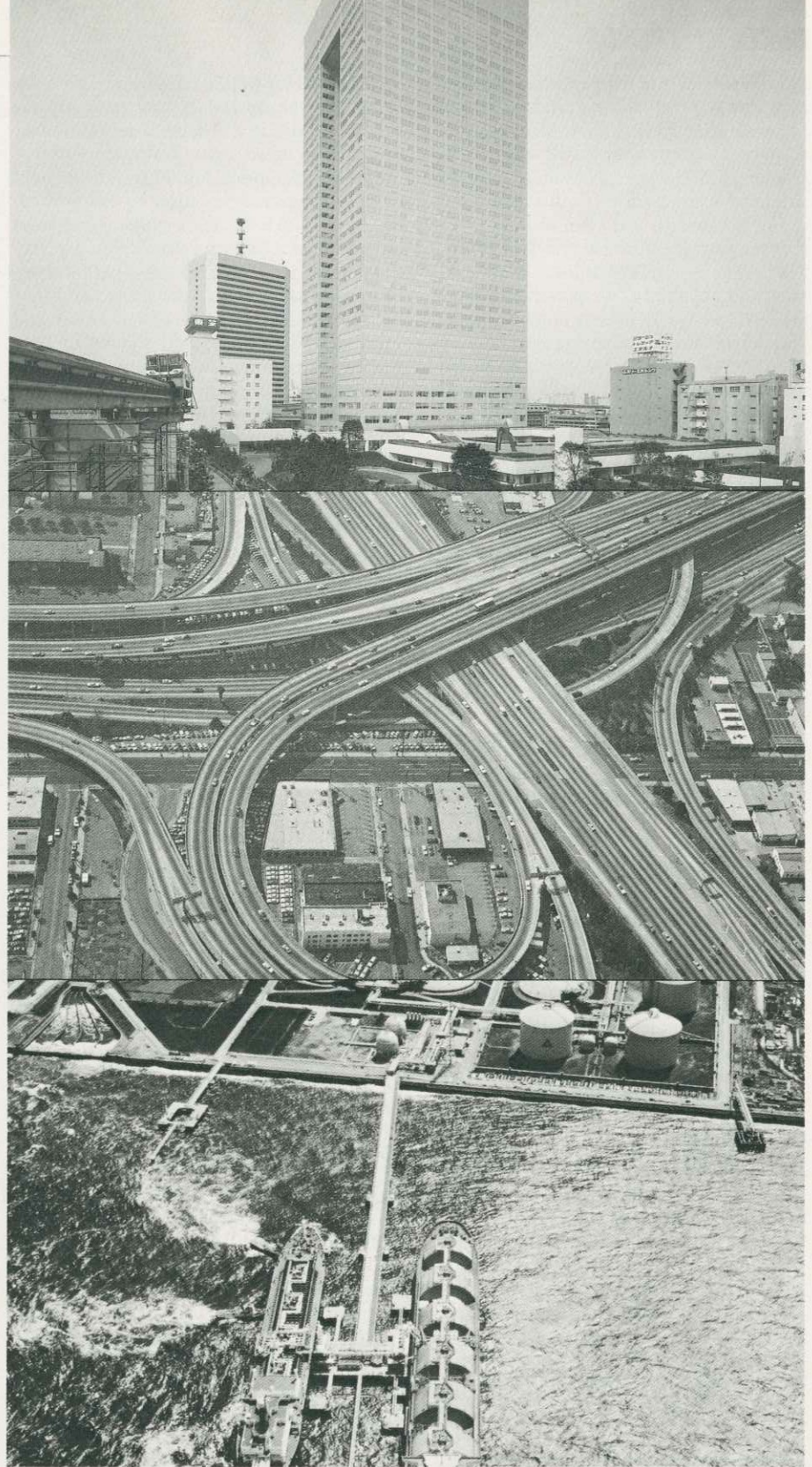
Optoelectronics technologies are widely used in building, expressway and sea transportation controls.
