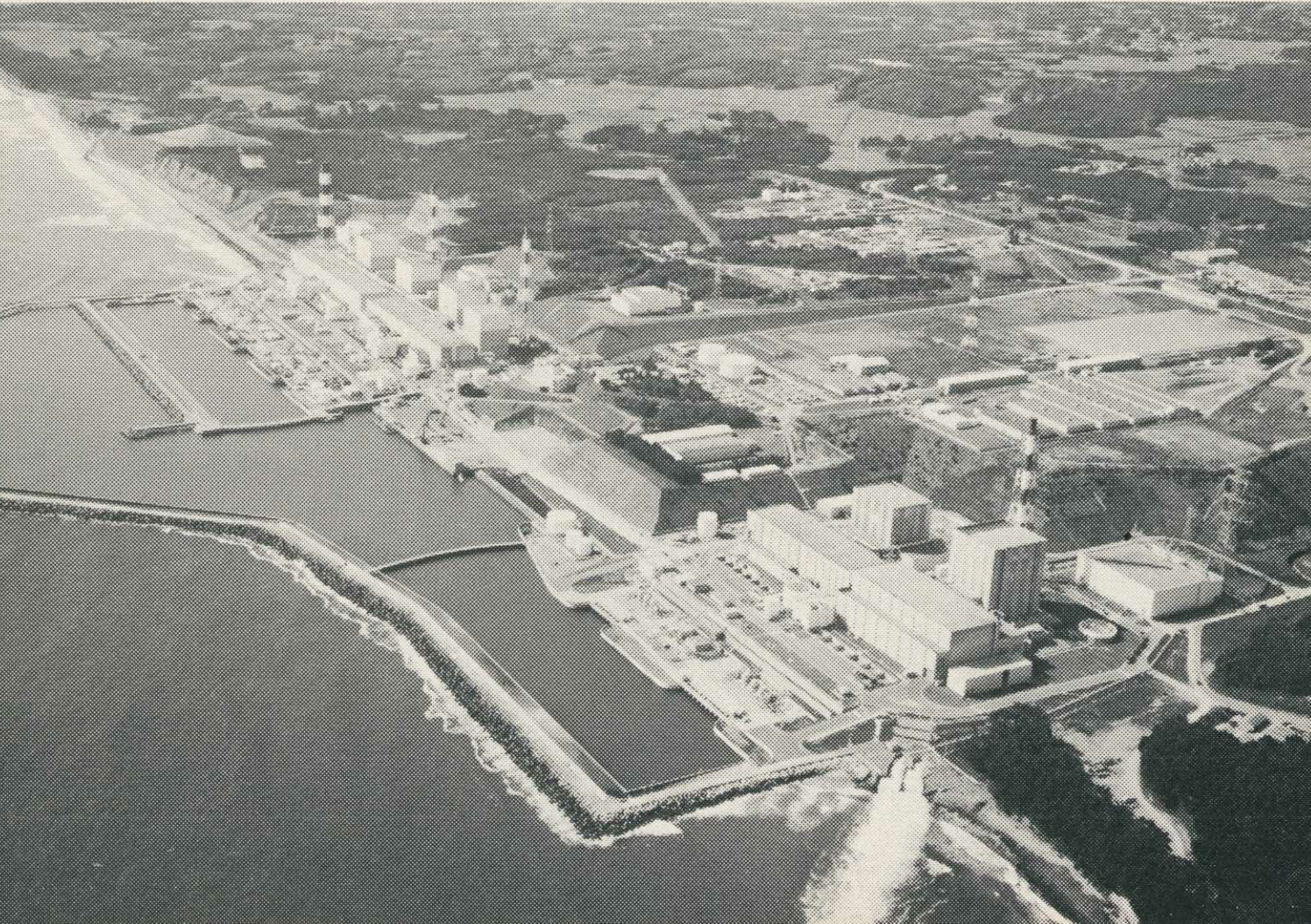
Nuclear power plant in Fukushima Pref. east of Tokyo
