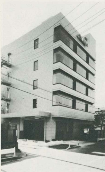
Molten Corp. headquarters in Hiroshima
