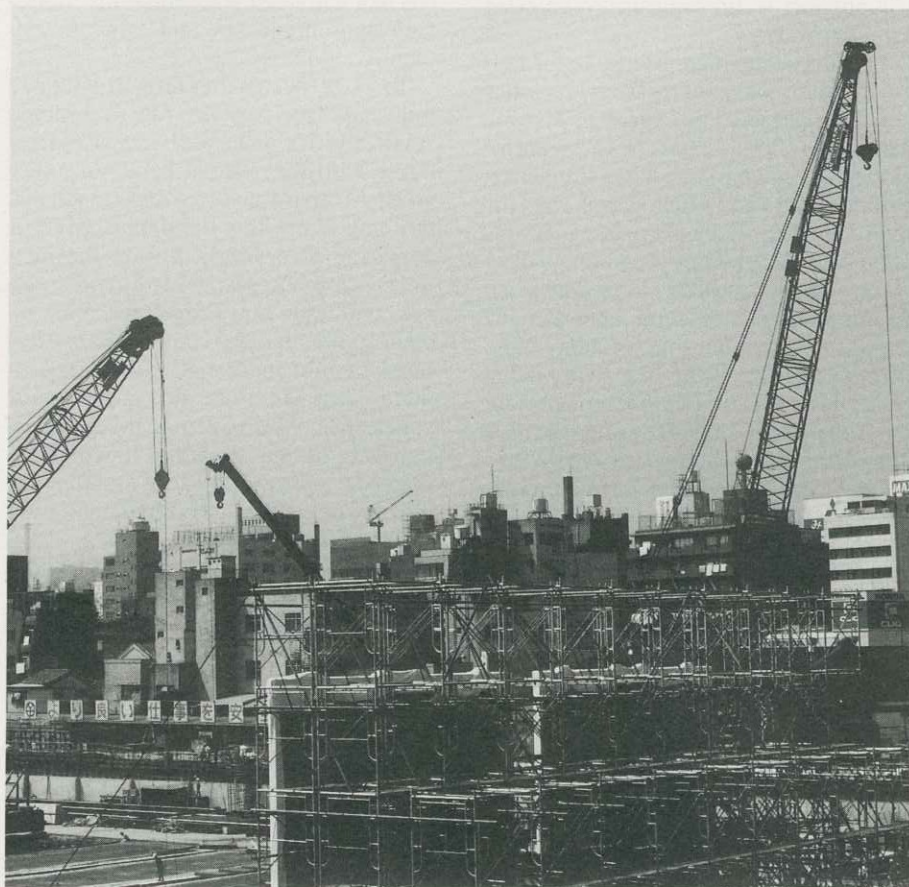
Housing construction and urban redevelopment are spearheading expansion of domestic demand.
